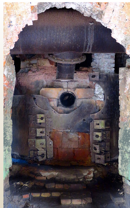
Remains of blast furnace in Bešlinec / Ostaci visoke peći u Bešlincu, References, notes (Reference, napomene)
